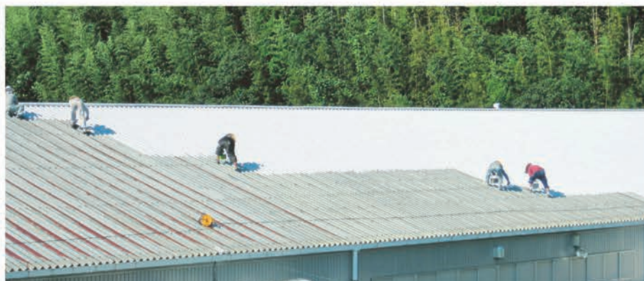
遮熱塗装工事 Heat-shielding paint application work
